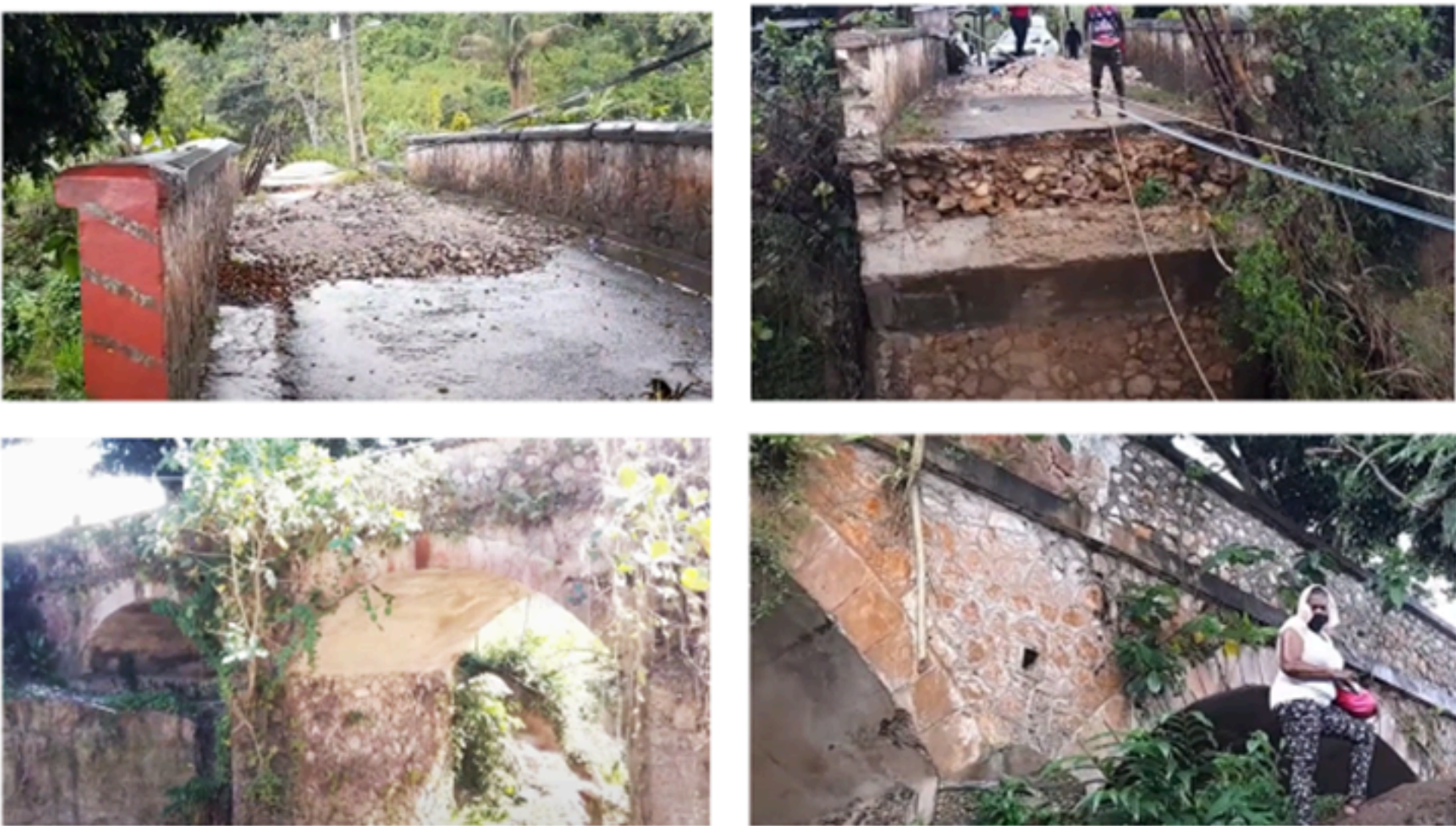
Figure 2. Images of the remnants of the bridge.
